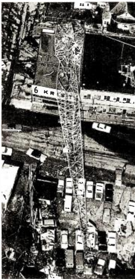
One of the first reports from the areas of the South devastated by Hurricane Celia last week was that the 145 mile-per-hour storm had flattened the tower of KRIS-TV Corpus Christi, Tex., knocking the station off the air. The structure was wrenched from its position on the roof of the station (top in photo) and strewn over the auto lot across the street. Communications with the storm-struck area were only partially restored by last Friday (Aug. 7) and no estimate of damages was available.
